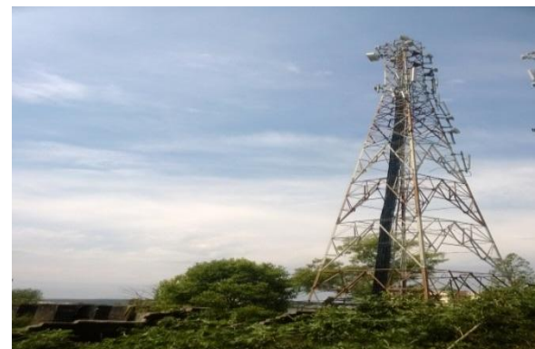
Fig.2 Radio signal base station along DIT-University, Dehradun.
