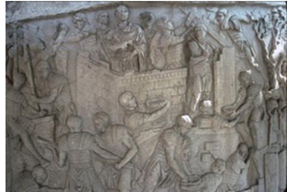
Figure 1. Roman soldiers building a fortress, Trajan's Column 113 AD ( http://en.wikipedia.org/wiki/Project_management )
