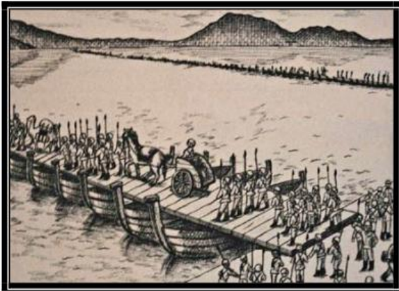
Fig.3 King Xerxes' Floating Boat Bridge across the Hellespont [2]
