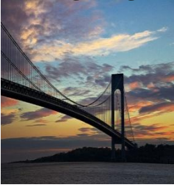
Original Annotation Bridge
