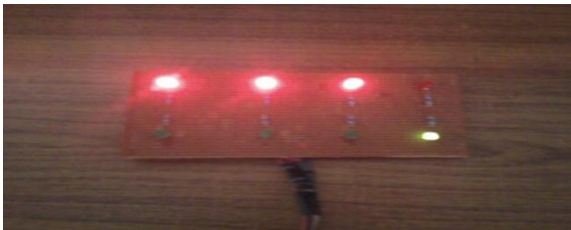
Fig 5.2: State of the tracking system at the control room when the train reached to station 1
