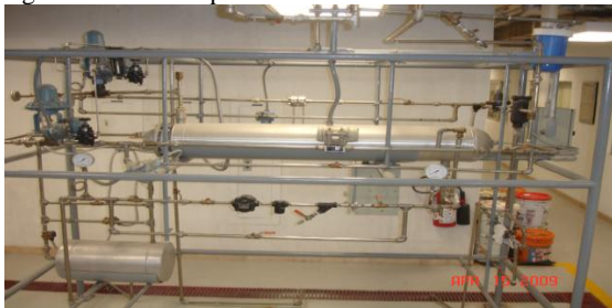
Fig. 7 Industrial heat exchanger used in the experiments
