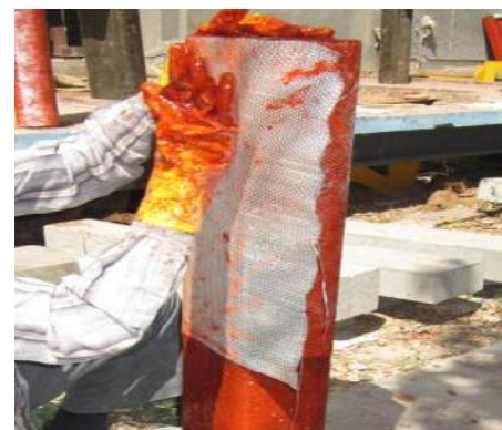
Fig.6 Application Of Gfrp Sheet
