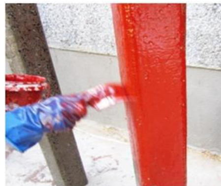
Fig.5 Application Of Saturant
