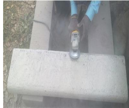
Fig.4 Grinding Of Rc Column
