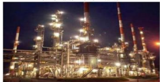
Fig 5. Smart Power Plants using LiFi
