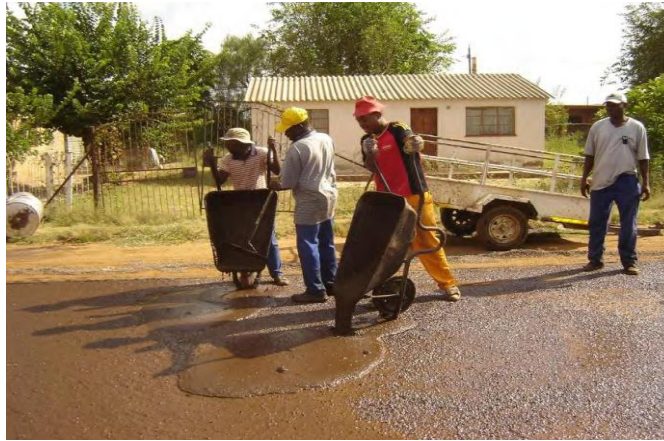
Fig 2: Placing of microsurfacing
