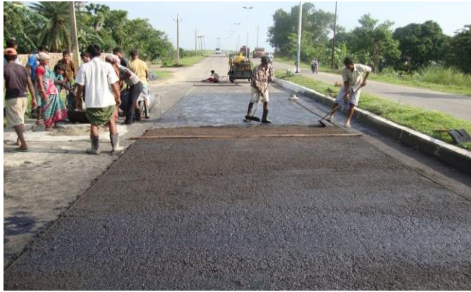
Fig 3. Microsurfacing at IIT-Guwahati approaching road
