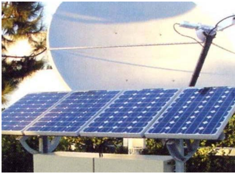
Figure 9: VSAT Equipment's powered by Solar
