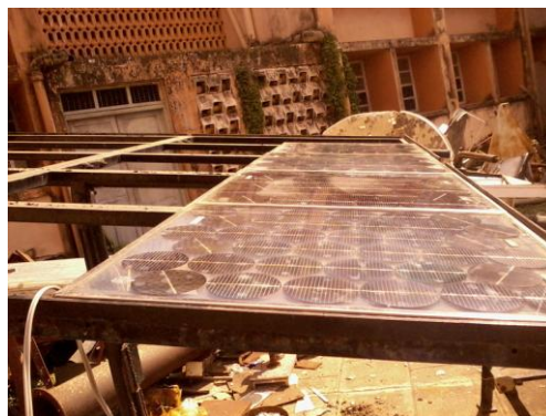
Fig 10(b): Solar Panel
